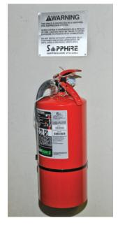
ANSUL SAPPHIRE cylinders contain 3M™ Novec™ 1230 Fire Protection Fluid for total flooding applications.
